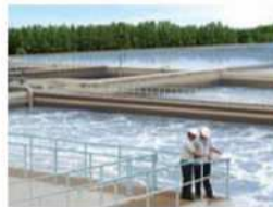
WATER TREATMENT SYSTEMS
